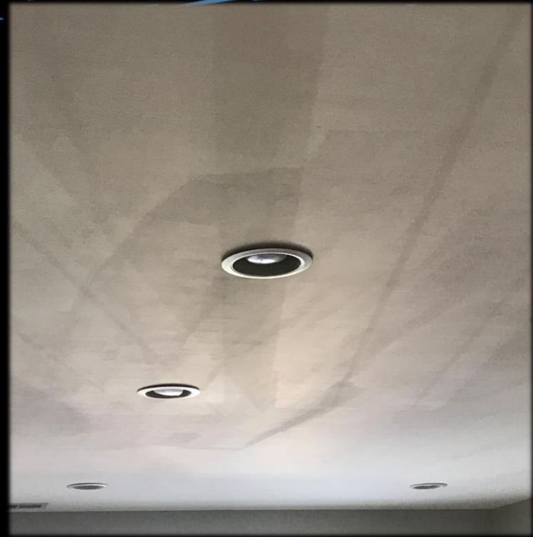
Shadows showing roller marks
