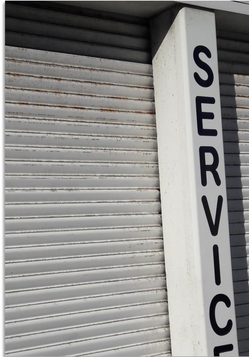
Sheltered from Rain Wash affect – Canopy Corrosion
