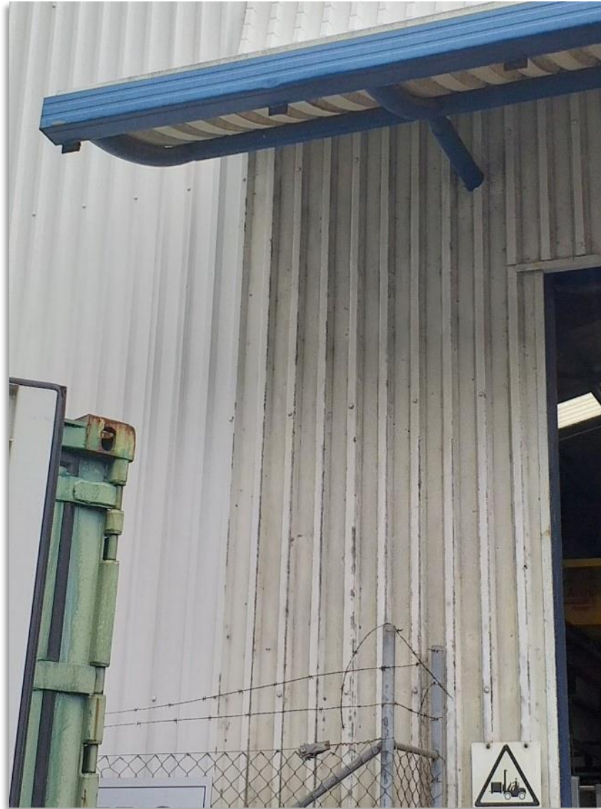
Sheltered from Rain Wash affect – Canopy Corrosion
