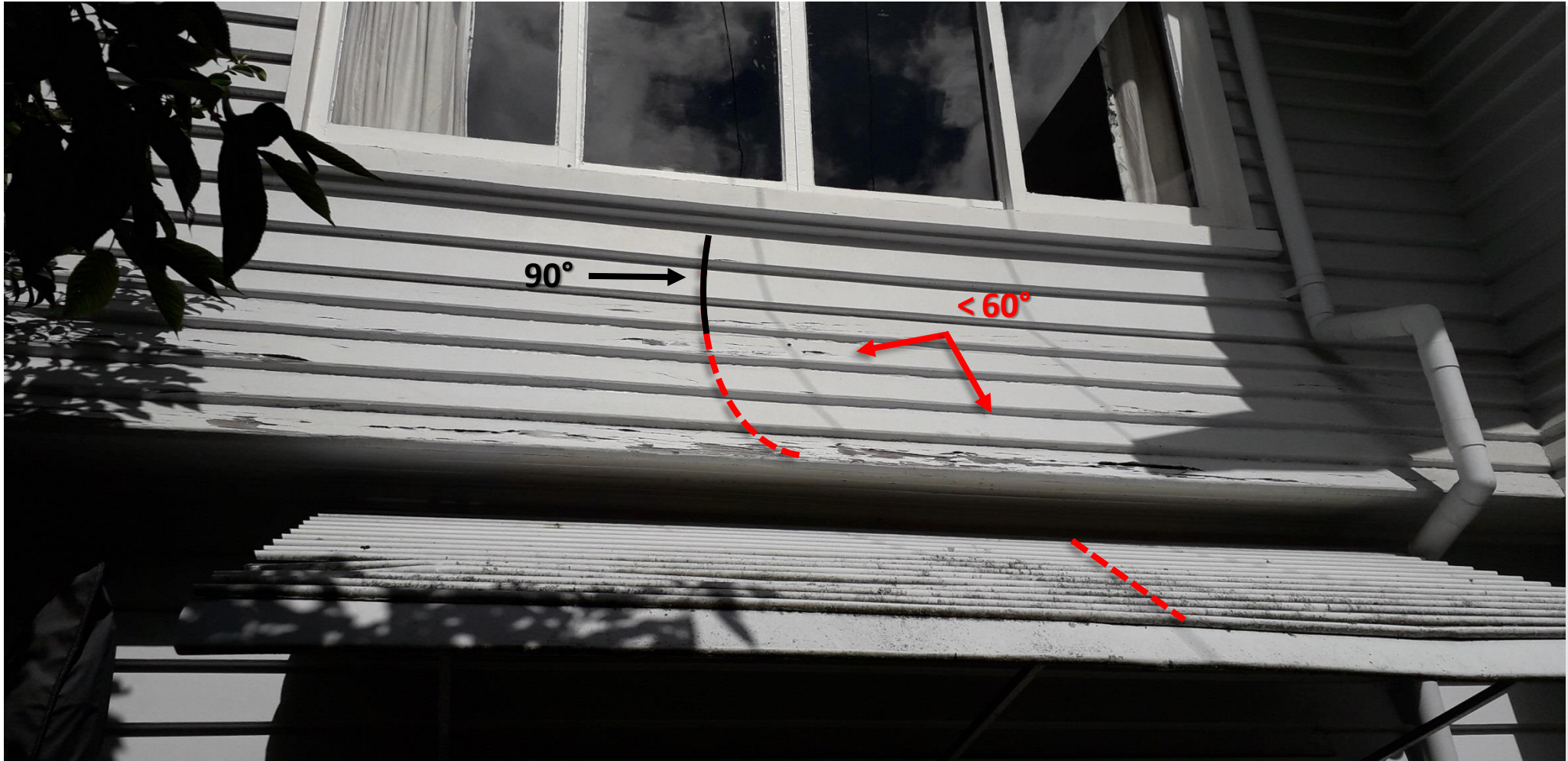
Affect of angle of exposure – an example of differential weathering
