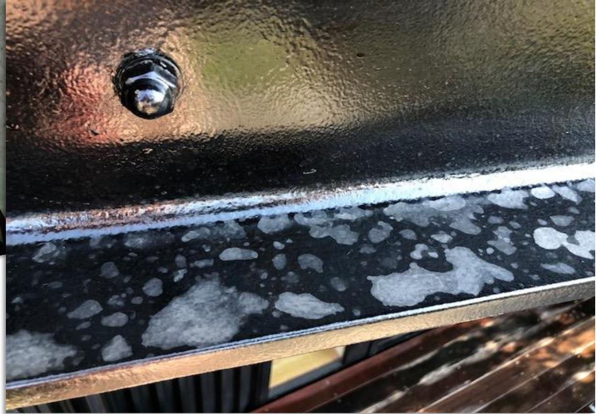
Effects of moisture / water on the surface of drying / curing paint
