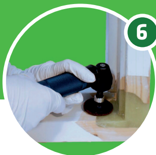
Sand finished repair
