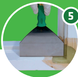
Shape and finish repair
