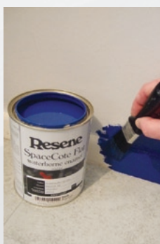
Step six Paint walls and skirting with two coats of Resene Decadence, allowing two hours for each coat to dry.
