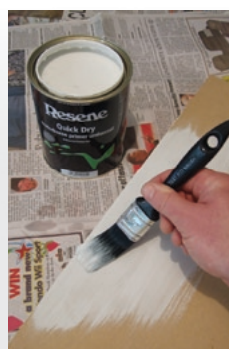
Step three Prime the MDF shelves with one coat of Resene Quick Dry and allow to dry for two hours.
