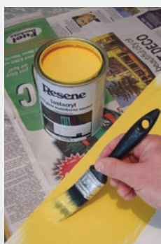
Step five Paint the shelves with two coats of Resene Supernova, allowing two hours for each coat to dry.
