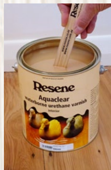
Step seven Carefully stir the Resene Aquaclear or Resene Qristal ClearFloor.
