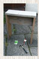
Turn the table the right way up and attach the table top to the legs and underneath support, fixing with nails and PVA glue. Punch in all the nail heads with the nail punch. Allow glue to dry.
