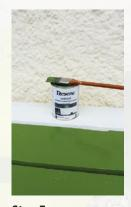
Step 7 Turn the bench the right way up and apply one coat of Resene Lustacryl tinted to Resene Green House to the top, sides and legs. Allow two hours to dry.
