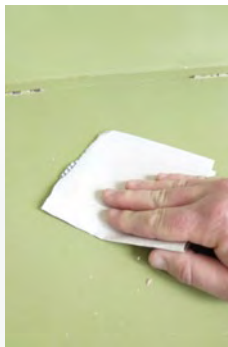
Step two Sand the filler smooth and then lightly sand the entire bench to 'key' the surface.
