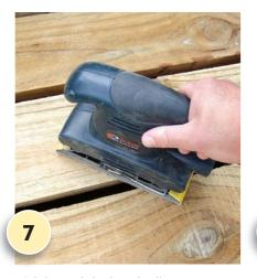
Lightly sand the boardwalk to ensure no splinters or rough edges remain.
