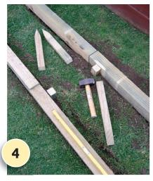
Bang pegs into the ground with the mallet at the ends and centre of each fence post, as shown. Then attach the pegs to the fence posts with two 100mm nails.
