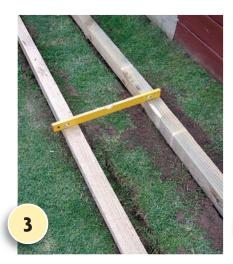
Lay fence posts in position, approximately 550mm apart. Dig two shallow channels to accommodate them. Ensure posts are level and the correct height for the finished path.
