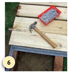
Nail each end of the fence paling lengths (stained side down) to the posts with two grooved decking nails. Use the 10mm piece of ply as a spacer between planks and the set square to keep planks at 90°.
