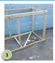
Measure and cut five 750mm lengths of battening and use to join side walls together, as shown, fixing at top and bottom with PVA glue and nails. Cut and fix two angled braces along the back wall.
