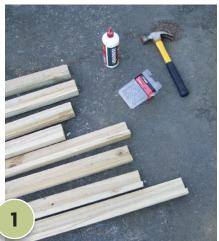
Measure and cut four 2m lengths and four 1.8m lengths of battening. Fix at right-angles with PVA and nails to create four rigid corner posts.
