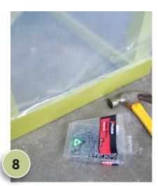
Staple PVC to the frame. Cut shade cloth to fit the front opening and staple at the top. Fix a length of battening to the bottom of the shade cloth. Attach two hanging brackets to hold the rolled shade cloth. Cut shelving from fence palings.
