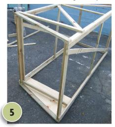
Cut two angled pieces of battening to fit across the roof pitch. Cut an angled piece of plywood to fit across the front panel's top to help to keep this panel rigid and square. Cut supports for the shelves and fix to side panels approximately 400mm apart.
