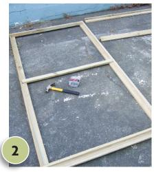
Fix four 1m lengths of battening at right-angles to create each rigid 'top' and 'bot-tom' support. Fix to the corner 'posts', as shown, to create a side wall frame. Fix the remaining 1m length 900mm from the bottom edge. Repeat for the second wall.
