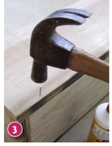
Fix the base into position, as shown, with PVA glue and 40mm nails. Allow glue to dry
