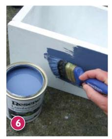
Apply two coats of Resene Astronaut to all surfaces of the window box, leaving two hours for each coat to
