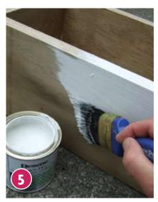
Apply one coat of Resene Quick Dry primer undercoat to all surfaces of the window box and leave to dry for one hour.
