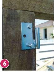
Fix the hinges to the gate and 100mm x 100mm post using the screws supplied (drill appropriate pilot holes first). Similarly, fix the latch to the gate and hang it.
