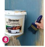
Apply a coat of Resene Pickled Bluewood to all timber surfaces, following the grain of the wood. Allow to dry for 24 hours before applying a second coat.
