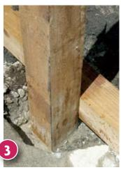
As in step one, concrete the two intermediate (100mm x 100mm) posts into the fenceline, allowing clearance for the gate to swing. Ensure all posts are the same height to accept two 75mm x 100mm top rails.
