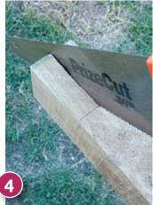
So the top rails accept each other at the corner, make a half-joint at each end of the two remaining lengths of 75mm x 100mm timber. Drill pilot holes and nail the rail (150mm nails) to the tops of the posts and the jointed ends at the corner posts.
