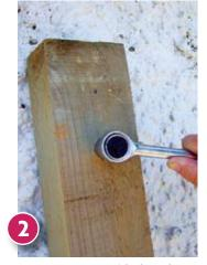
Repeat step one with the other 75mm x 100mm end-post. If your walls are solid concrete, as with this garage, use dynabolts to help secure the post. Drill into the concrete with a 12mm masonry bit. Ensure the three dynabolts are countersunk into the post. Tighten with a ratchet.
