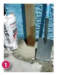
Dig a hole 60cm deep, hard up against the house. Position one 75mm x 100mm end-post (as shown) and fix into position with a bag of quickset concrete, following manufacturer's instructions.
