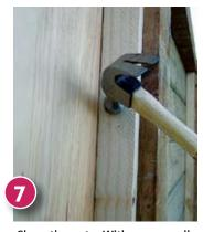
Close the gate. With 50mm nails fix 25mm x 50mm battens to the posts around the gate so it butts up, ensuring a neat finish. Repeat along the top edge of the gate then attach the remaining battens along the upper edge of t&g cladding.
