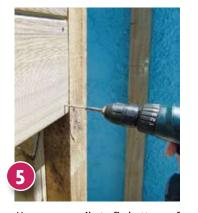
Use 75mm nails to fix battens of 50mm x 50mm timber to the post sides (inset approx 15mm from the front edge). Measure and cut the tongue and groove (t&g) to fit between the posts. Working from the top down, drill the t&g and screw it to the 50mm x somm battens.
