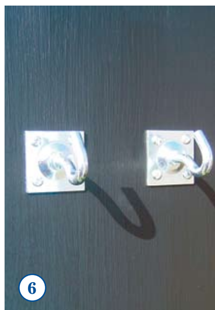
6 SCREW the washing-line hooks into position.
