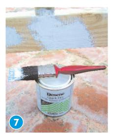
HANG the gate on the hinge supports and check that it is level (if not, adjust the hinge supports by lightly tapping one further into the pillar with a hammer). Apply one coat of Resene Quick Dry Acrylic Primer Undercoat to the gate, and allow to dry.
