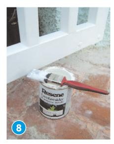
APPLY two coats of Resene Alabaster to the gate, leaving two hours to dry between coats. Drill a 10mm hole in the other pillar and fix the galvanised latch to the gate, ensuring the latch is aligned with the hole in the pillar.
