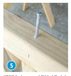
USING the long 5mm drill bit, drill a hole through the outer frame and into each of the 50mm x 50mm railings. Insert a 150mm galvanised nail into each of these holes and gently tap into position with a hammer.
