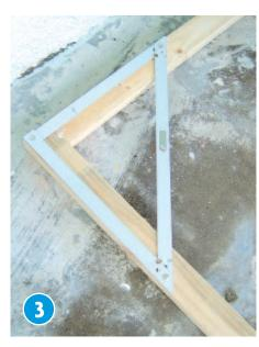
PLACE the frame on a flat surface and use the large set square to ensure the corners are at accurate right angles.
