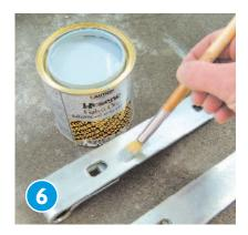
APPLY one coat of Resene Galvo One to the hinges. Once dry, fix the hinges to the gate with galvanised coach bolts and fix the hinge supports into the pillar using a 10mm masonry drill bit and strong exterior construction glue (use a spirit level to check that they are perfectly aligned).
