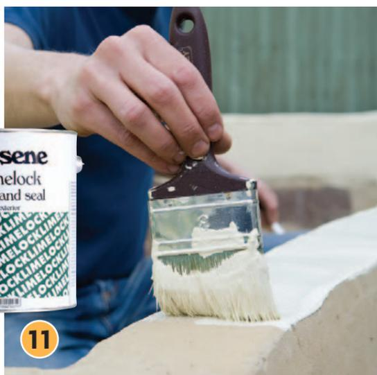
**11** If using Resene Lumbersider in a dark, heat-absorbing colour, leave the Limelock a week before painting over. Otherwise leave for a day and paint two to three coats of Resene White (or other pale colour). Resene Limelock's ability to cure and seal the concrete eliminates the need to leave it to cure for seven days before painting.
