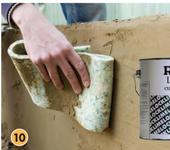
**10** Before the second coat goes off completely, gently rub it with a piece of foam or sponge. This will smooth out imperfections and give the plaster a consistent finish over the whole surface. Then immediately apply a coat of Resene Limelock and allow to dry. Apply a coat of Mulseal Plus waterproofing membrane to the inside of the bed to prevent water coming through the blocks and affecting the paint.
