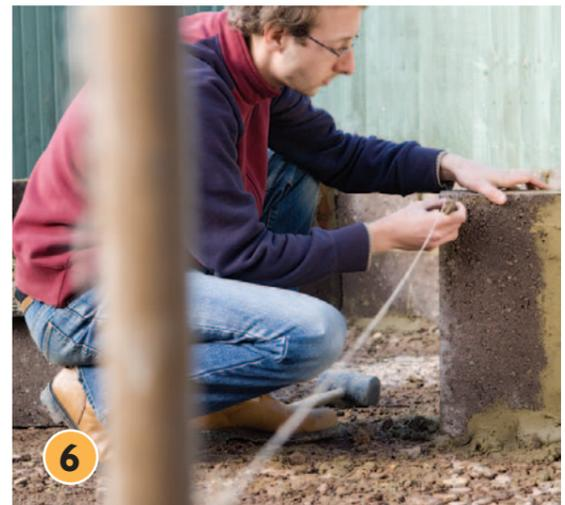
**6** When it comes to making the curved edges of the bed, lay concrete blocks on their short ends (this is the exact height of the two blocks on top of each other used for the straight edges). This time, use a bed of mortar that is roughly 5cm deep. It's important to keep checking that the curved line matches up to the mark on the string tied to the pole.
