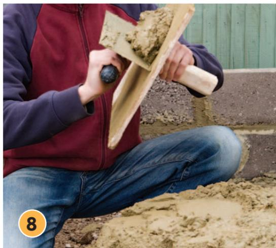
**8** Mix a mortar of five parts sand to one of cement, enough to fill the cavities in the blocks. Fill them and hose lightly, ensuring the top of the second course of blocks has an even finish. Allow to go off. Once set, make a plaster (render) mix of three parts sand to one part cement. Add a dash of washing-up liquid as a plasticiser to make the mix smoother and easier to apply. Mix to a creamy consistency.
