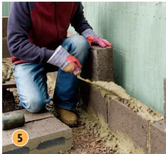
**5** Lay the second course of concrete blocks on top of the first, using another bed of mortar, this time about 2cm deep. Make sure the two layers form a brickwork pattern, using a hammer and bolster chisel to cut blocks in half for the ends. Check the levels again.
