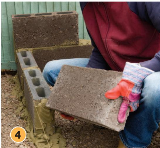
**4** Mix a mortar of five parts builders' sand to one part cement. It's easiest to use a cement mixer, especially if you're building a large bed. Starting with the sprayed straight edges, lay the first course of blocks, placing them on their longest end, on a bed of mortar 5cm deep. Run a length of string between two pegs to help keep the blocks in a straight line. Use a spirit level to check the blocks are level.
