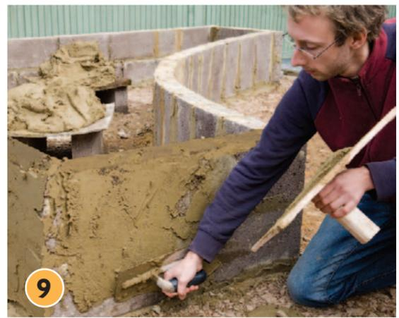
**9** Apply the first coat of plaster to the blocks. It should be 5-10mm deep and it doesn't matter if it's quite crude. Cover the outside. You'll only need to plaster halfway down the inside of the bed, as the soil will cover the rest. Once you've finished, score large diamond patterns into the surface using the corner of your trowel. This is called a scratch coat. Wait for the scratch coat to go off overnight, then apply a second, smoother coat on top. Don't worry if the finish is a bit rough.
