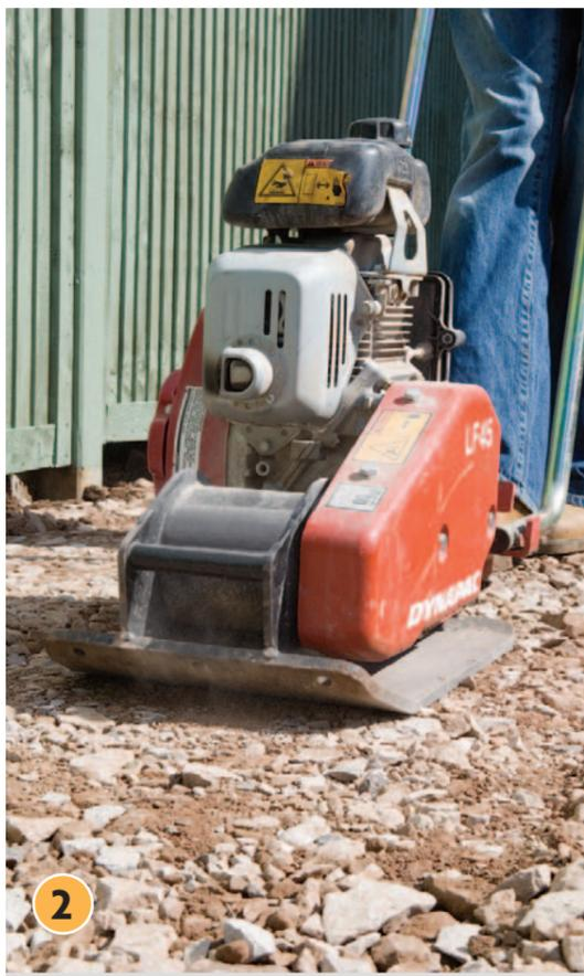
2 Compact the basecourse using the plate compactor to a uniform dense condition. This will ensure the footings for the bed are more secure.
