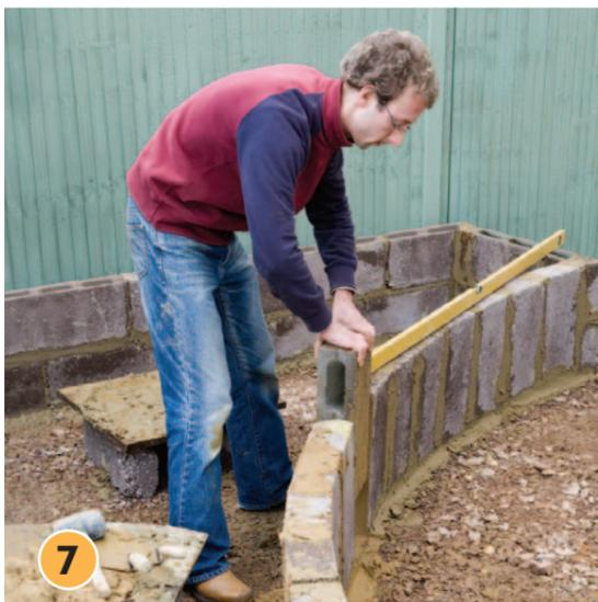
**7** Lay the ends of the curved edges first, working in towards the centre. Carefully slot in the last block, cutting it to size if necessary. Make sure all edges of the bed are level on the vertical and horizontal, and tap them straight with a rubber mallet if necessary. Leave the whole thing to go off (set) overnight.
