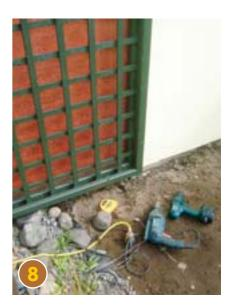
USING a drill, screwdriver and copper screws, attach the 1.8m square capping frame to the garage wall, and screw the trellis panel to the square capping frame.
