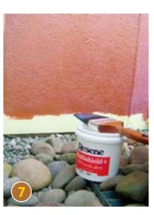
USING a paint roller, apply two coats of Resene Enamacryl in Resene Copper Fire to the 1.75m square. Allow to dry and finish off with one coat of Resene Multishield+ Gloss.
