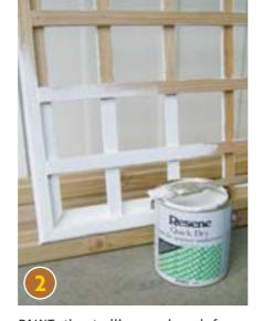
PAINT the trellis panel and fence capping with one coat of Resene Quick Dry Acrylic Primer Undercoat. Allow to dry.
