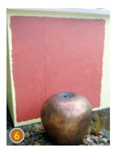
USING a large brush and "stippling" technique, apply a generous coat of Resene Sandtex in Resene El Salva, covering the 1.75m square. Allow to
