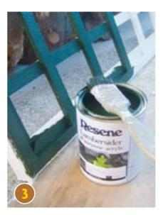
PAINT the trellis and fence capping with two coats of Resene Black Forest, allowing two hours to dry between
