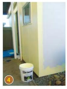
PAINT the garage walls with two coats of Resene Pale Prim, leaving a 1.75m square where the trellis will be attached.
