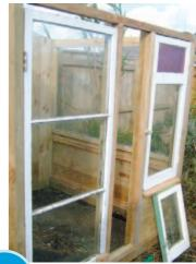
Hang the hinged front window and door and fix inner upright framing on the front wall using four 25mm x 50mm battens. Construct lower section of front wall (under window) using remaining fence palings and create an angled sill from an offcut of fence paling. On the side wall create a glazing frame from the 25mm x 50mm battens and fix the glass pane into place and hold with silicon sealer and 20mm x 20mm moulding.
