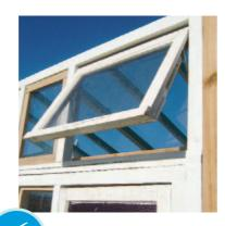
Fix the two hinged windows within the upper frame and create a fixed central window using the 25mm x 50mm battens. Using 25mm x 50mm battens, create three fixed windows down the centre of the front wall panel. Measure and have glass cut to fit and hold in position with silicon and 20mm x 20mm moulding. Fit the remaining four 25mm x 50mm roofing battens.
