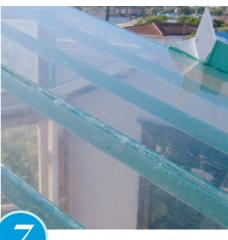
Using 25mm x 50mm battens, create two triangular side windows - one in line with the pitch of the shed roof, the other with the pitch of the glasshouse roof. Glaze these, supporting the glass with 20mm x 20mm moulding and silicon sealer. Fix safety glass panels to roof with silicon sealer and hold in position with nails supporting lower edge.
