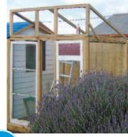
Using 50mm x 50mm battens, construct the upper front window frames, supporting the structure with central and end roof battens as shown. Prime roof battens with one coat of Resene Quick Dry Acrylic Primer Undercoat, and finish with two coats of Resene Patina.
