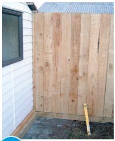
Against the side wall of the shed, create a level square base with the four 100mm x 100mm fence posts. On a flat surface, construct the rear wall panel from five 50mm x 50mm fence battens and 12 fence palings using galvanised nails and exterior wood glue. Fix the rear wall panel into upright position, nailing through the timber base and shed wall
