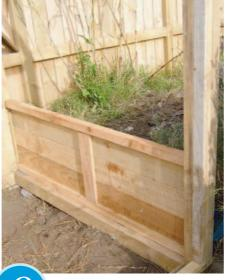
Using galvanised nails and exterior glue, construct the low side wall using three horizontal fence panels and 50mm x 50mm battens and fix four upright 50mm x 50mm battens at the front corner (as shown). Fix a 50mm x 50mm batten along the lower front edge of the wooden base frame.
