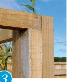
Using galvanised nails and glue, fix an upright 50mm x 50mm batten at the other front corner (nailed directly to the shed wall), fix one 50mm x 50mm batten along the top edge of the front wall and another along the top edge of the side wall (as shown).
