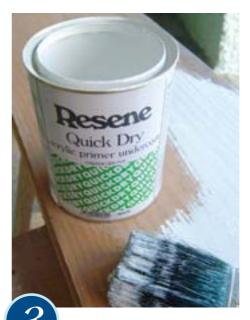
PRIME the seat planks with one coat of Resene Quick Dry Acrylic Primer Undercoat. Prime all the edges and ends of the paling dividers and base plinths.
