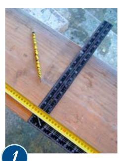
WITH the tape measure, pencil and set square, mark the 300mm x 50mm timber into five 900mm lengths, then cut to size with the skilsaw. This will form the seat.
