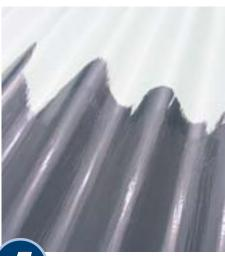
WHEN dry, apply two coats of Resene Lumbersider tinted to Resene Ebony Clay on both sides of the iron panels. Alternatively, use Resene Hi-Glo in Resene Ebony Clay for a glossy finish.
