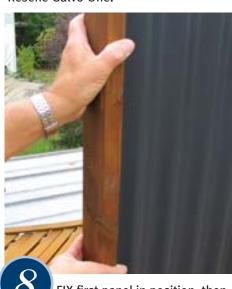
FIX first panel in position, then fix remaining panels to one another with fence fastenings, one at the top and bottom of each panel.
