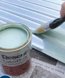
APPLY a coat of Resene Galvo-Prime to the iron panels. We've used new corrugated iron sheets. If using weathered sheets, prime with Resene Galvo One.
