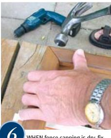
WHEN fence capping is dry, fix mitred corners with galvanised nails or screws. Leave one end of the frame open. Some adhesive on the mitred joints will make for a better connection.
