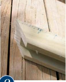
TO make the frames, measure the iron sheets then cut four corresponding lengths of fence capping for each panel (2 sides, 1 top and 1 bottom), cutting ends at a 45° angle.
