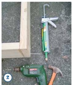
CONSTRUCT a square base frame from the four lengths of timber using glue and nails. Fill any imperfections with exterior filler. Once set, sand and prime with Resene Quick Dry Acrylic Primer Undercoat, then paint with two coats of Resene Deep Koamaru.
