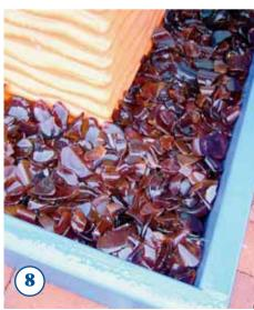
TOUCH up any damage to paint and apply one coat of Multishield+ gloss to base frame. Once dry, cover the plastic trellis with a layer of smooth bottle glass or pumice. Turn on the water pump and enjoy!
