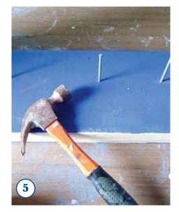
HAMMER a level row of galvanised nails along each inner edge of the frame, then attach black polythene to the frame using flathead galvanised nails.
