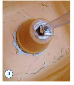
MIX Knead It adhesive according to manufacturer's instructions and glue the small terracotta pot over the hole on inside base of the remaining large terracotta pot. Use bricks to hold in position until Knead It dries (about an hour).
