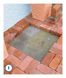
SWEEP existing concrete and lay reclaimed bricks in a basket weave pattern, leaving a square gap, as shown. Position two of the large terracotta planters against the wall.
