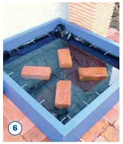
LAY the frame with the plastic lining over the gap in the bricks and fill with water. Position four bricks and stand terracotta pot upside down in the centre of water feature's base.
