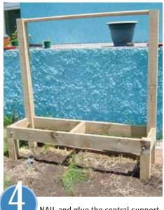
NAIL and glue the central support beam. Temporarily position top length of fence capping to ensure the seat is set square and level.
