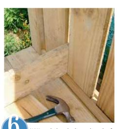
NAIL and glue the lower length of fence capping along the back of the seat and slide the fence palings into position between the upper and lower lengths of fence capping, ensuring they're evenly spaced. Fix the top fence capping to the top of the rear legs with glue and nails.
