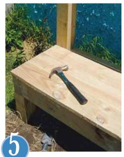
NAIL and glue three fence palings to form the seat. Cut a fourth paling to fit along the back edge.
