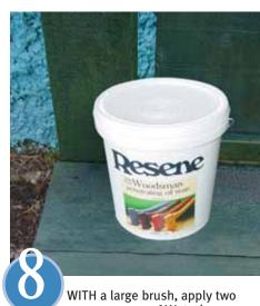
generous coats of Waterborne Woodsman oil stain tinted to Resene Rangitoto. Allow to dry, then plant two vines of the grape 'Schuyler' at either end of the bench and attach to the back palings with plastic coated wire.
