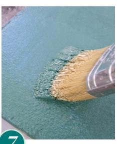
ONCE cured, the concrete step should be diamond ground or acid etched (see note above). Paint with Resene Non-Skid Deck & Path.
