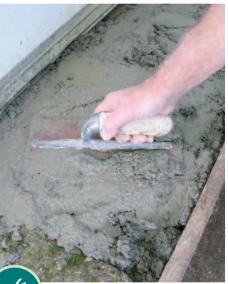
FILL the frame with the concrete, using a trowel. Work the concrete in and out with the trowel to compact the mix and eliminate air pockets.
