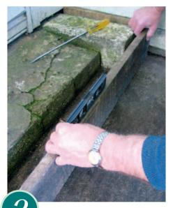
INSTEAD of removing the old step, we've concreted over the top. Build a frame out of the wood scraps around the old step.
