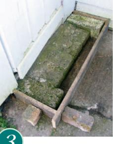
NAIL the frame together and brace firmly with concrete blocks or wooden braces. Use a level to ensure the frame is straight. Mix the concrete.
