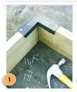
Use the 4 DIY garden corners to attach one 1.2m fence paling across the top of the two 1.5m fence palings, fixing them into position with 30mm galvanised nails, as shown.
