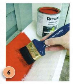
Apply two coats of Resene Red Berry to the entire unit and allow two hours for each coat to dry. Position the unit against a fence or wall and secure with the two angle brackets.
