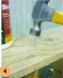
Align the back edge of each shelf with the pencil marks. Angle each shelf at about 45° and fix in place with PVA and 50mm nails. Stand the unit upright.
