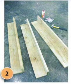
Fix the six remaining fence palings together at right angles to form the three shelves, as shown, using 50mm galvanised nails and PVA glue.
