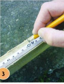
Measure down from the top of the unit, and make three pencil marks along each side about 400mm apart.
