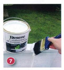
Apply two coats of Resene Alabaster to the entire cold frame and the window frames, allowing two hours for each coat to dry. Firmly fix the clear plastic to the underside of the window frames using 25mm nails or galvanised staples.
