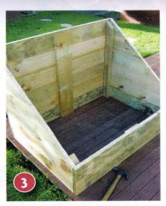
Assemble the main body of the cold frame using 40mm nails and PVA glue.
