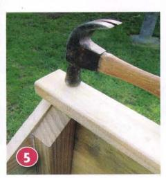
Fix one 1200mm length of fence capping along the upper edge of the cold frame, using 40mm nails and PVA glue. Repeat with the second length of fence capping along the lower edge.
