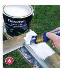
Apply one coat of Resene Quick Dry primer undercoat to the entire cold frame and also to the window frames. Leave to dry for one hour.
