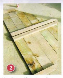
Form the two side panels, as shown, using the 800mm lengths of fence paling and the lengths of 50mm x 75mm timber - note how the upper ends are cut at angles to follow the pitch of the sides. Again, fix with 40mm nails and PVA glue. Leave to dry - preferably overnight.
