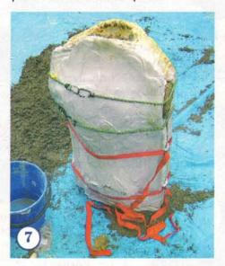
SECURE the mould with ties, plug the arm holes with clay, then fill with concrete. Once dry, use warm, soapy water to remove the mould. Sand or fill any imperfections with cement.
