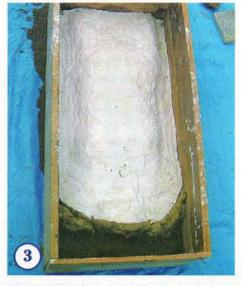
COVER the mannequin, clay and plywood with a generous layer of petroleum jelly and build up several layers of casting plaster to a thickness of 40mm.
