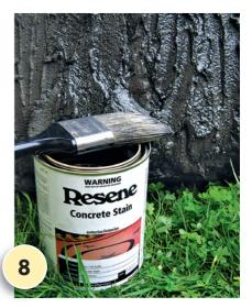
After 28 days, once the concrete has fully cured, apply two coats of Resene Concrete Stain Black to the cat, allowing four hours for each coat to dry.
