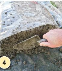
Mix a slightly drier concrete mix and fill the base of the mould, as shown, levelling off with the trowel.
