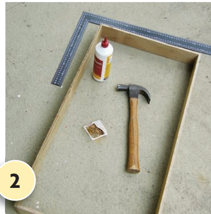
2 Assemble the tray's sides, forming a 785mm x 420mm rectangle. Fix at each corner with PVA glue and panel pins (remember to drill pilot holes first). Use a set square to make sure corners are at right angles.
