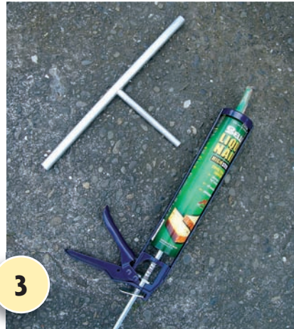
3 Cut a 350mm length of 16mm tubing and a 135mm length of 12mm tubing. Drill a 12mm hole at the mid-point on the 16mm tubing. Slide the 12mm tubing into this hole to form a 'T' shape and fix it with construction glue.
