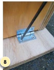
Fix two hinges to the front wall's top edge and roof, leaving an about 50mm overhang. Fold the underfelt in half and place in the box.
