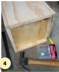
Position the floor approximately 30mm from the bottom edge, as shown, fixing it in place with PVA and nails.
