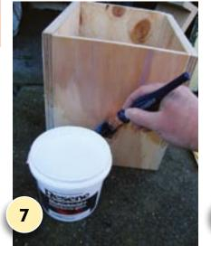
Apply three coats of Resene Multishield+ gloss to the box's exterior surfaces and roof, allowing two hours for each coat to dry.
