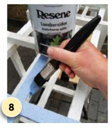
Apply two coats of Resene Time Out to the frame, allowing two hours for each coat to dry
