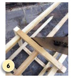
Trim the bottom off both central vertical supports, as shown. Ensure the cut is flush with the edge of the bottom strut. Leave the frame overnight for the glue to dry.
