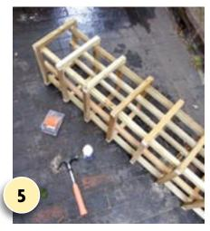
Using the same technique, join the front and back sections together with eight horizontal struts down each side – align these side struts with the struts on the front and back.
