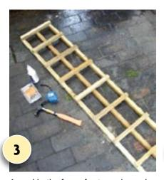
Assemble the frame front, as shown, by fixing eight horizontal struts about 160mm apart with plenty of glue and nails (drill pilot holes first). Use a set square so corners are at right angles.
