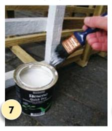
Apply one coat of Resene Quick Dry to the frame. Allow two hours drying time.
