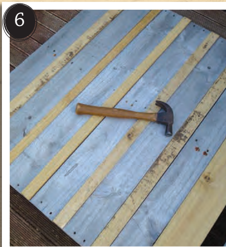
Turn the planter over and fix the bases from the back using 50mm nails.
