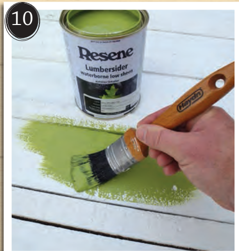
Apply two coats of Resene Koru to the entire planter, allowing two hours for each coat to dry. Place the planter in position, fill each section of the planter with good quality potting mix and plant up with potted colour.
