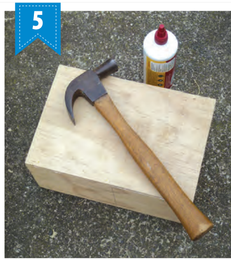
Attach the base to the box, fixing with PVA glue and 25mm nails.
