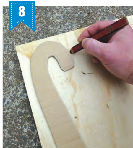
Place the template on a piece of 9mm plywood and trace around the edge, as shown. Reposition the template and trace a second handle.
