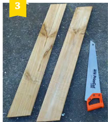
Repeat steps one and two to create two fence palings with angled ends, as shown. These will form the sloping sides of the display ladder.
