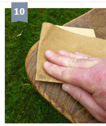
Lightly sand the filler and wipe off any sanding dust with a clean cloth.
