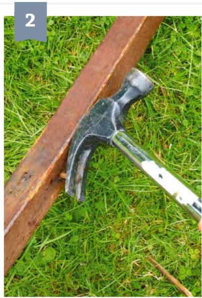
Remove any nails using a claw head hammer. Again, take care not to damage the wood.
