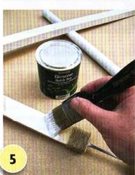
Apply one coat of Resene Quick Dry to the wooden cross piece and the smaller wooden top piece, as shown. Leave to dry for two hours.
