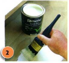
After leaving the unit overnight for glue to dry, drill three or four drainage holes in the box base. Then apply one coat of Resene Quick Dry to the entire unit. Allow this and all other coats of paint used in this project two hours to dry.
