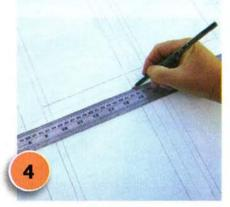
Mark the 'window and shutters', making shutters 200mm and outer window frames and glazing bars 35mm wide. Mark 10mm 'shadow' strips along bottom of the top and horizontal glazing bars and on the right of the left and vertical bars.
