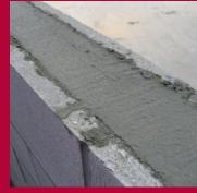
PaintCrete after being levelled off at the top surface of the wall.
