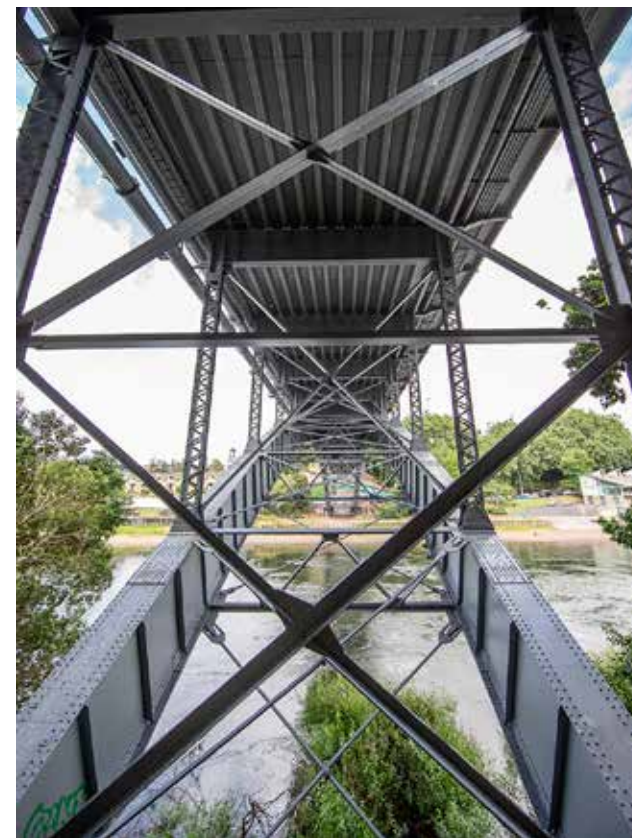
above: Hamilton's Victoria Bridge is coated in Altex Coatings Haze Grey.
