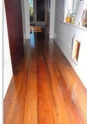
Typical gloss of coatings is quoted at the 60° angle however the 85° angle is also good to know, as it helps to indicate side sheen affect, especially relevant for long hallways (as in the photo example above).
