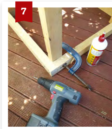
Using PVA glue and 75mm screws, fix the 450mm lengths of timber at each corner of the frame to form table legs, as shown. Clamp firmly while the pilot holes are drilled and screws put in position.
