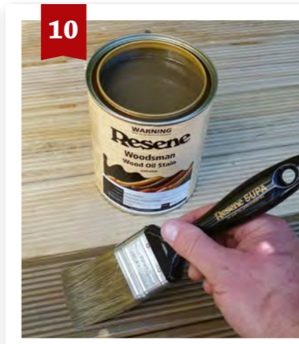
Apply two coats of Resene Woodsman to the table allowing 24 hours for each coat to dry.
